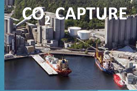
Norcem HeidelbergCement Cement plant
