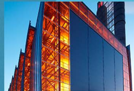
Oslo City Waste-to-energy plant
