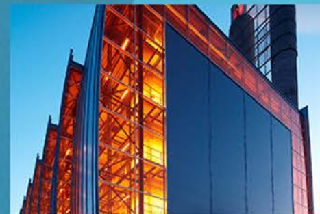
Oslo City Waste-to-energy plant
