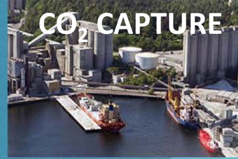
Norcem HeidelbergCement Cement plant
